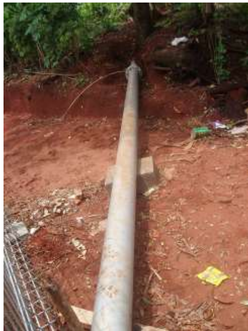
Gambar 2. Pipa Besi Distribusi
