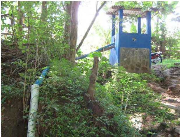
**Gambar 2. Pipa Intake Ke Pompa**
